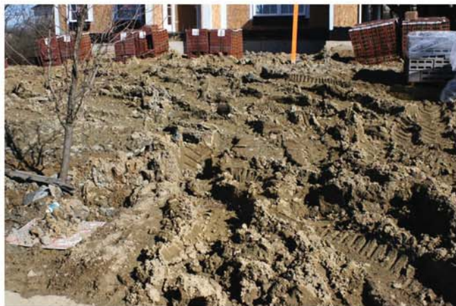
Figure 5 - Although compaction causes serious damage to the soil, it leaves behind all of the preexisting soil horizons; the organic layer and topsoil have just been squeezed down.
