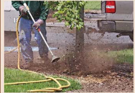
Figure 10 - An air knife removes soil from a tree root zone without damaging the roots. The technique is generally reserved for small trees due to the risk of making larger trees unstable.
