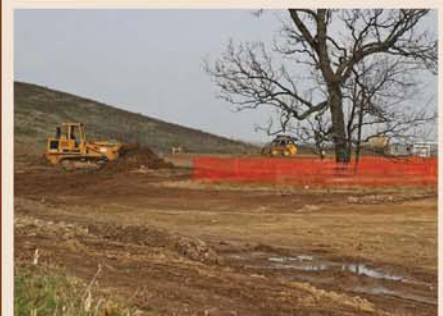
Figure 12 - A CRZ—critical root zone—should be created around mature trees to keep construction equipment from compacting the soil near established roots.
